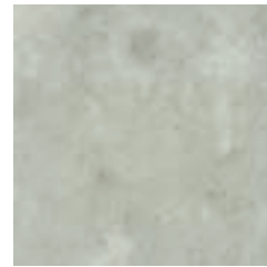
Worn Concrete TL39 S
