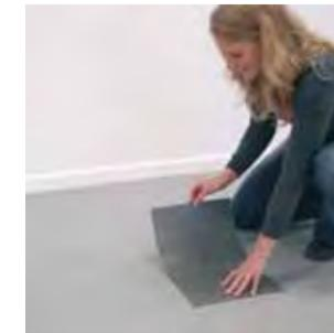
5. Install the first plank or tile from this central point.
