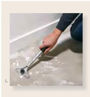
1. Before laying, the base must be clean, hard, smooth and dry.
