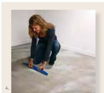
4. Establish the centre of the room by drawing two perpendicular lines on the floor.
